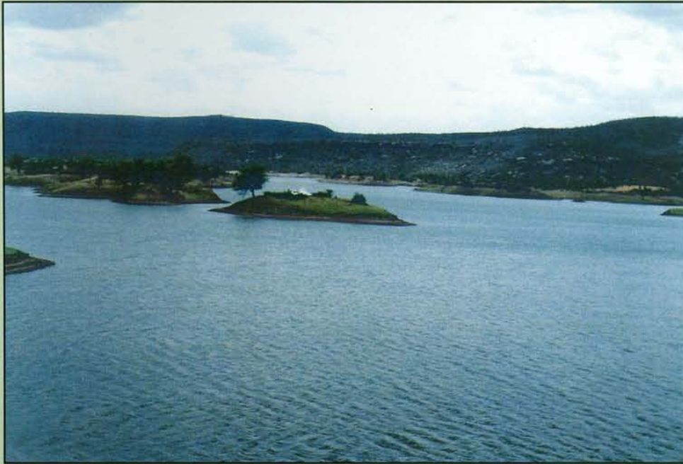
Fig. 25 A view of Needar Reservoir
